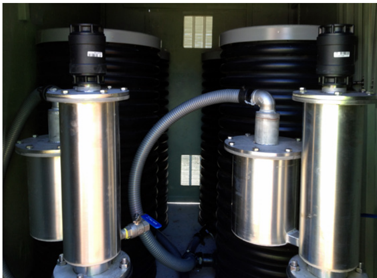
VS-4-S with emergency vacuum air flow orifice of 1900mm 2 Odour control elimination shown
